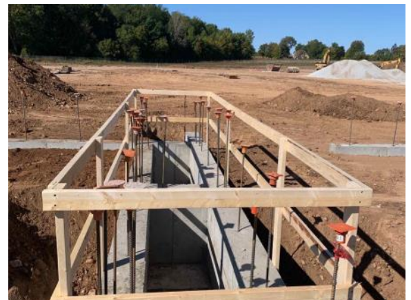
Completed concrete footing section (9/28/2021)
