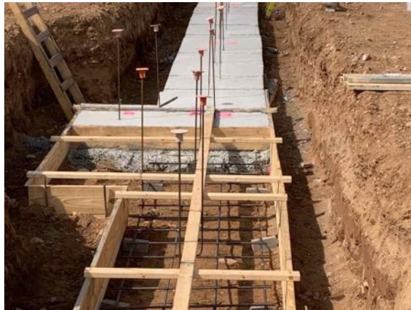
Concrete footing with rebar reinforcement (9/13/2021)
