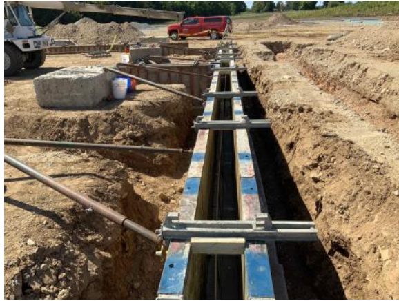
Concrete foundation wall forms (9/1/2021)
