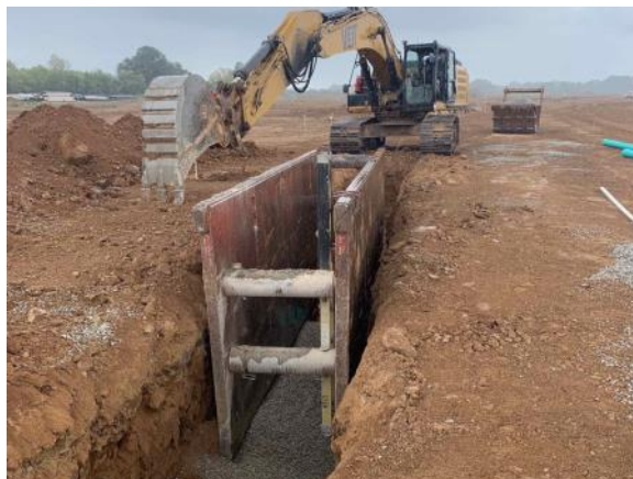
Water main installation (9/20/2021)
