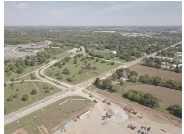
Aerial view of road closure (9/17/2021)
