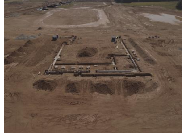
Aerial view of concrete foundations in the future gym (9/7/2021)
