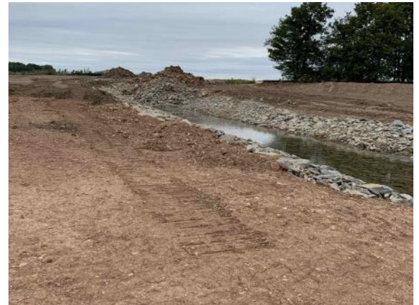
Future inlet to storm retention pond (9/13/2021)
