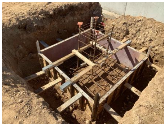
Concrete column pad formed and ready to be poured (9/15/2021)
