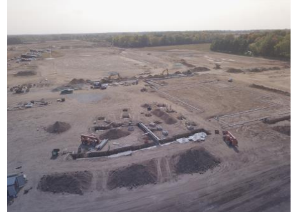
Concrete footings in future orchestra/choir rooms (9/30/2021)
