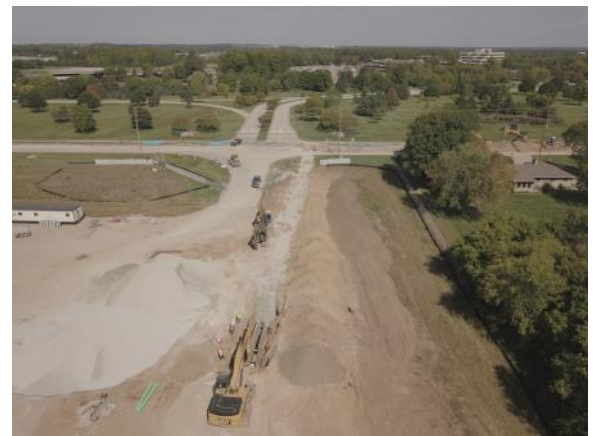
Sanitary sewer installation near main entrance from Hwy II (9/17/2021)
