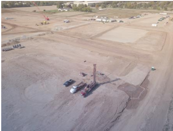
Well drilling for geothermal field begins (9/30/2021)
