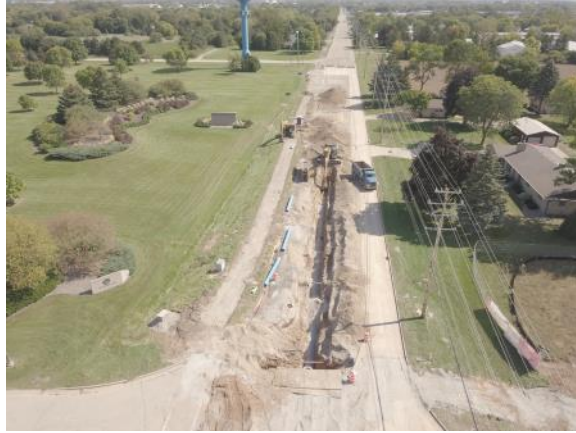
Water main installation in County Hwy II (9/17/2021)
